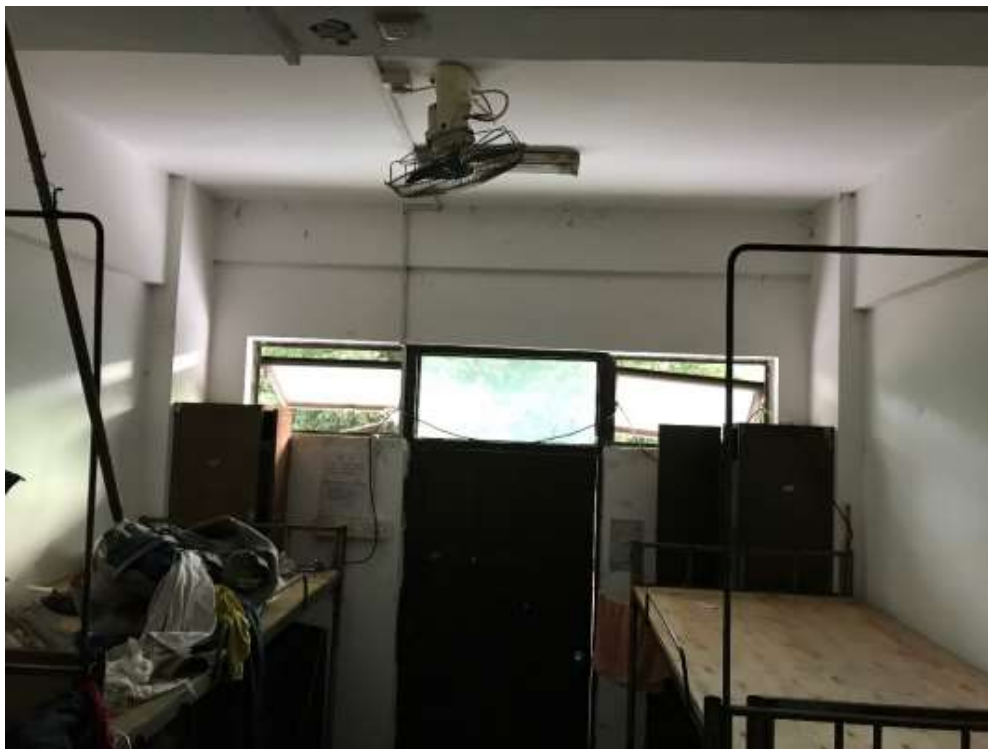
Interior of the dorm room, only two fans were installed in the room
