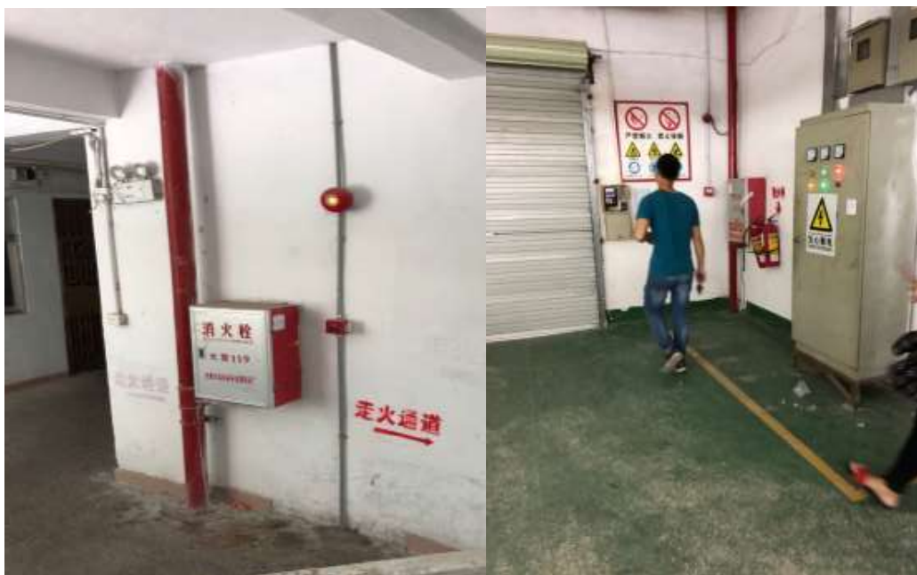
Left: fire hydrant and sign indicating where the emergency escape route is; Right: fire hydrant and fire extinguishers in the workshop as well as signage prohibiting smoking
