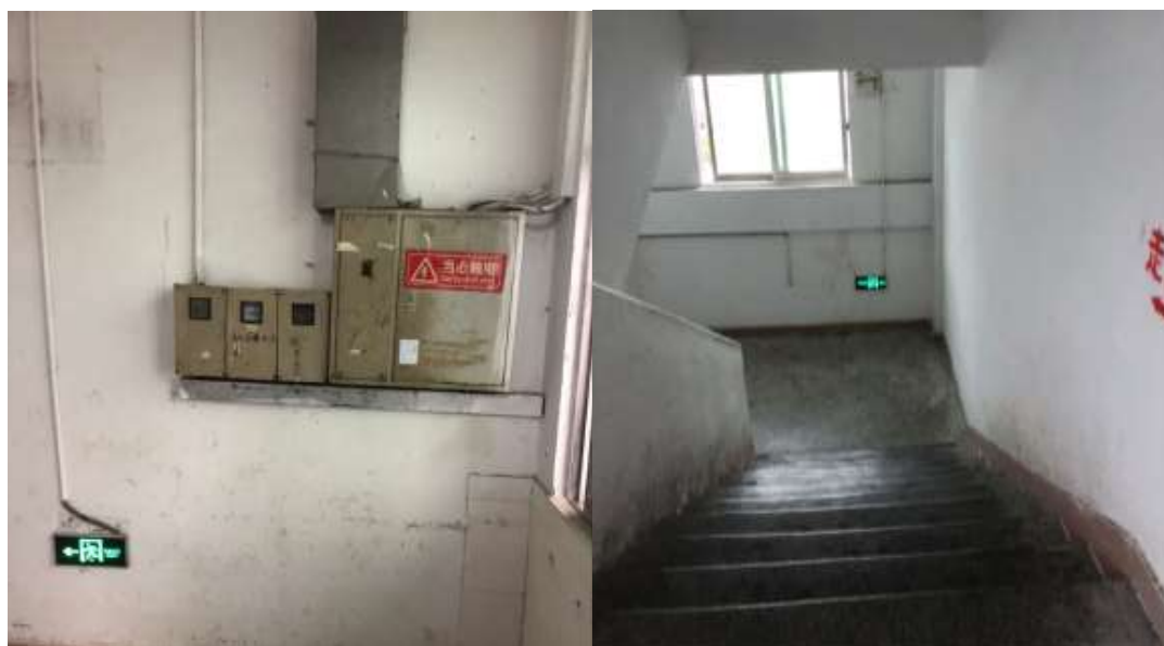
Emergency exit signs
