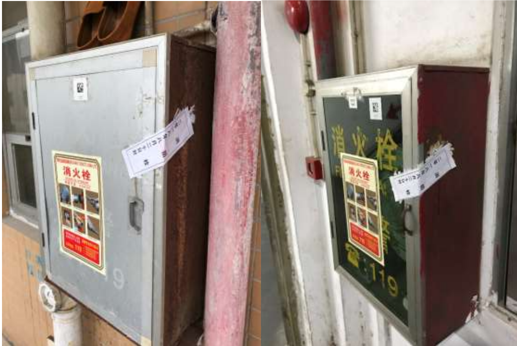
The fire hydrants in both the dorm and workshop had inspection log on it
