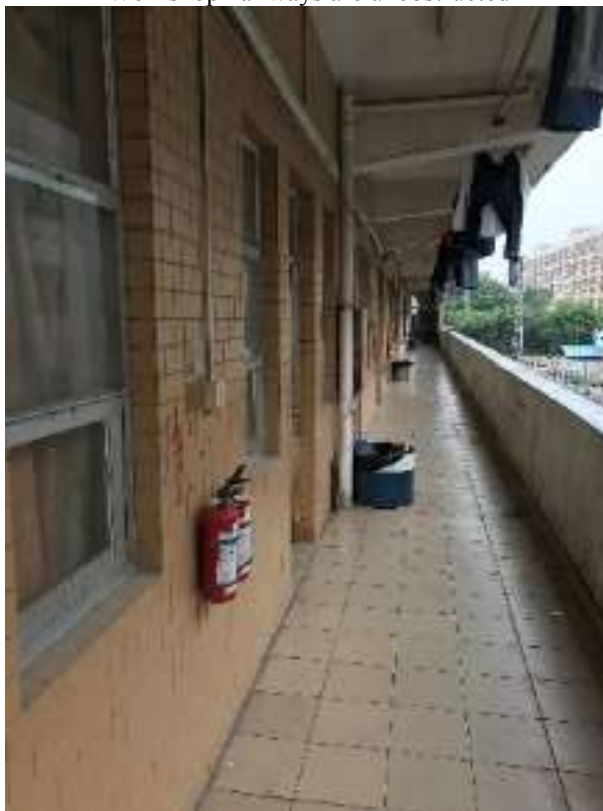
Dorm hallway is unobstructed
