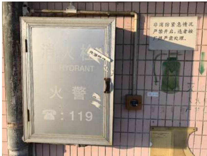
Fire extinguisher and fire hydrant
