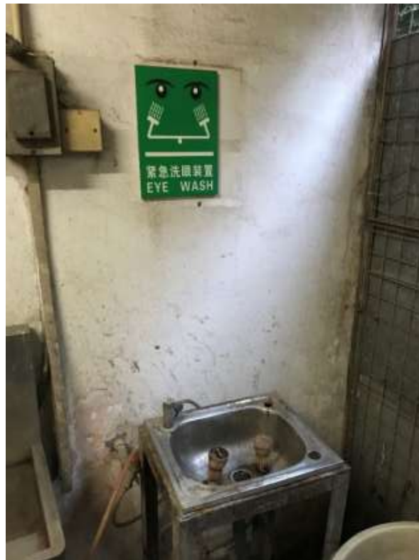
Emergency eyewash station
